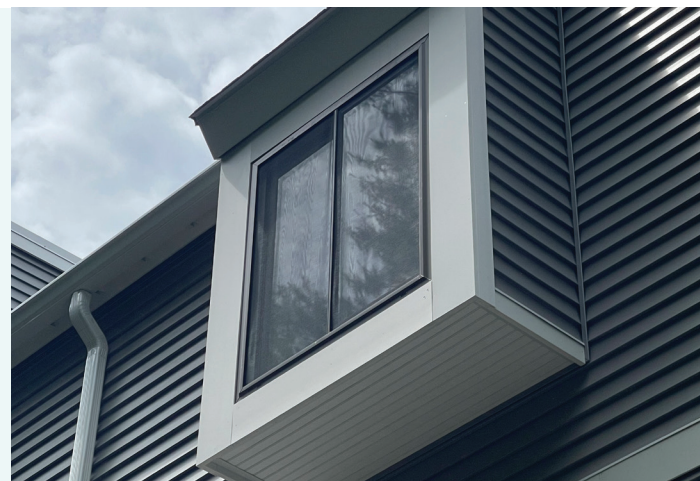
Photo: Completed window enclosure
