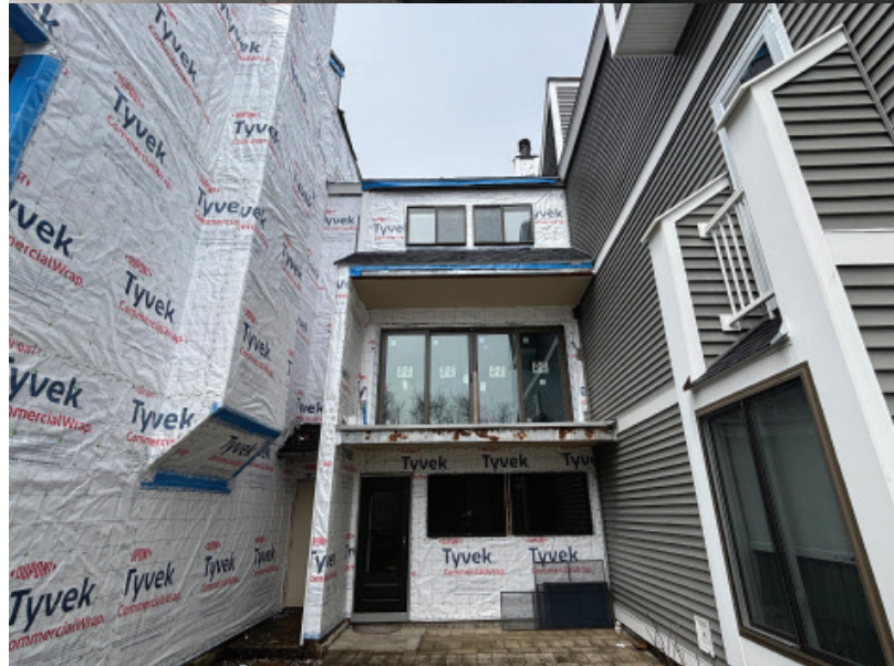
Photos: Pre and mid construction
